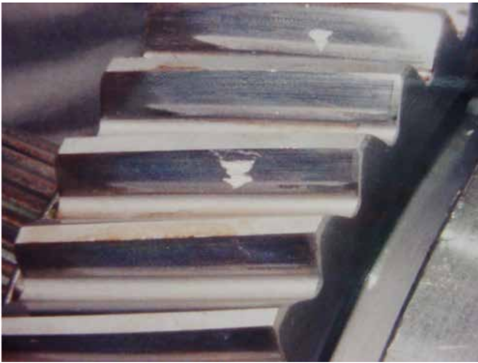
Figure 6: Inclusion initiated pitting in vacuum degassed steel.
